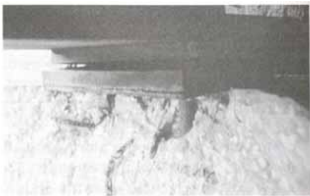
Exhibit XII.1 Fracture of Bearing Seat
